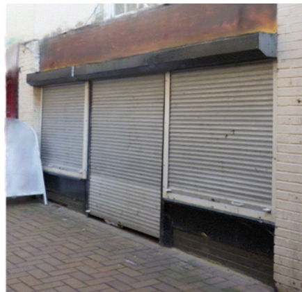
Photograph showing closed or solid grill which provides a negative image.
