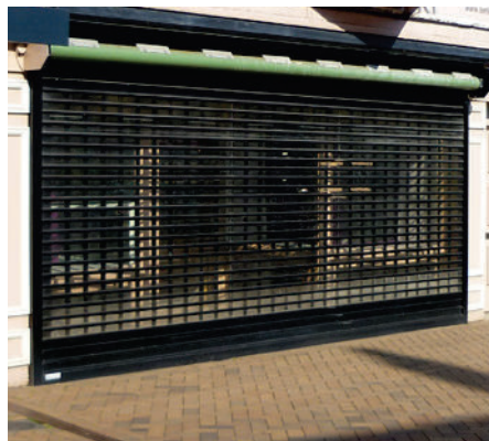
Photograph showing open grill which does not close the active frontage and provides security.
